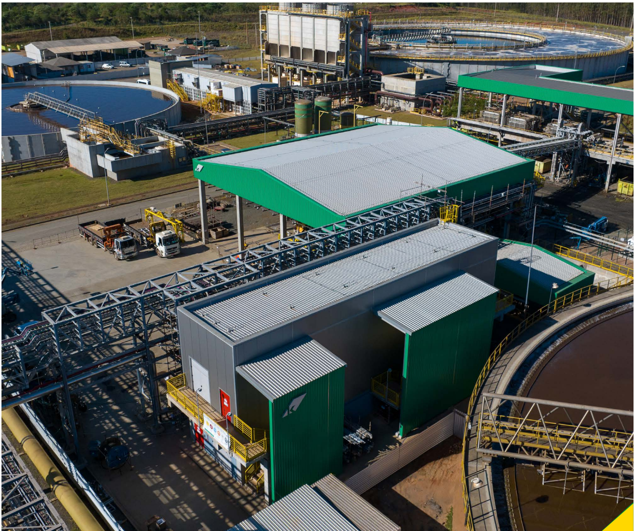
Sludge drying plant in Ortigueira (Paraná)
